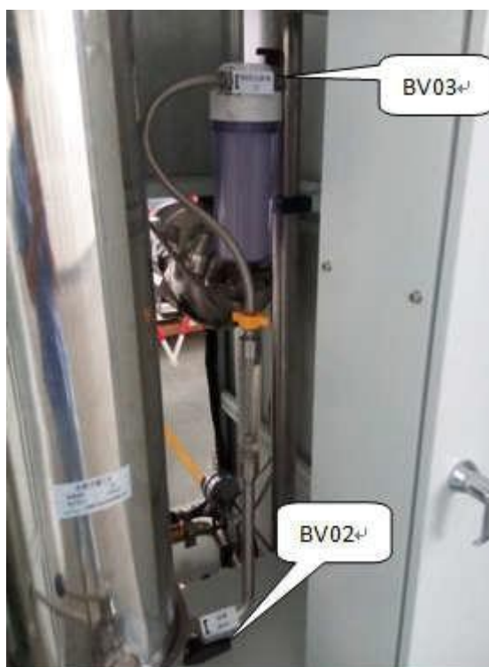
图 8.7 滤芯 Z2 示意图 Figure 8.7 Schematic diagram of filter element Z2
